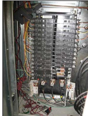
**FIGURE 2-4 – LIGHTING PANEL HA WITH MONITORING EQUIPMENT**
